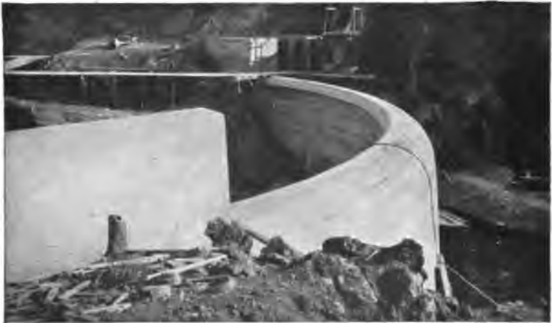
FIG. 243.—Diversion Dam, East Park Feed Canal, Orland Project.
